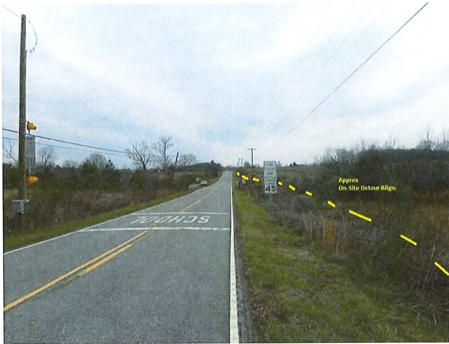
Photo 2.1 Facing east towards bridge showing approximate lay-out of temporary on-site detour.
